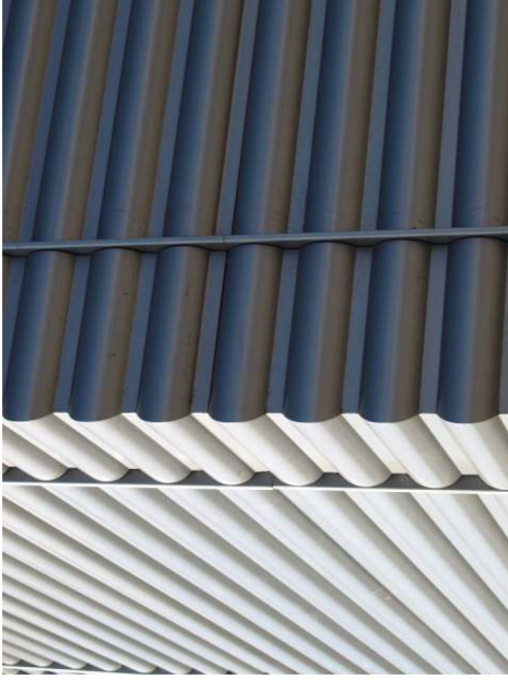
DETAIL 2 Mitred external corner to half round profile cladding
