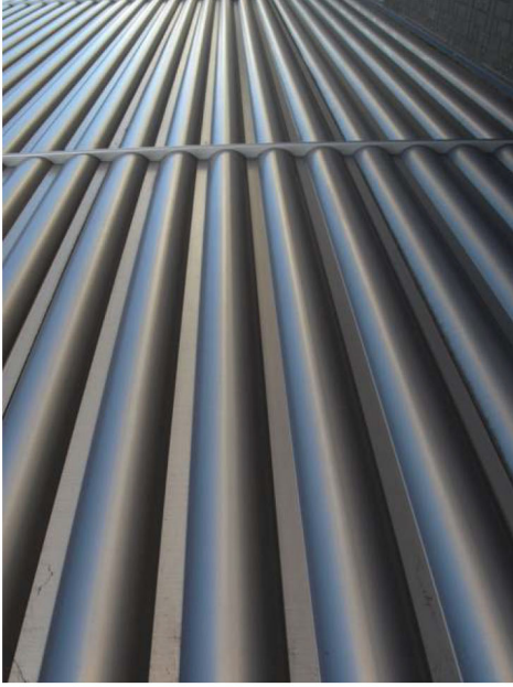
DETAIL 3 Vertical finger flashing in contrast colour
