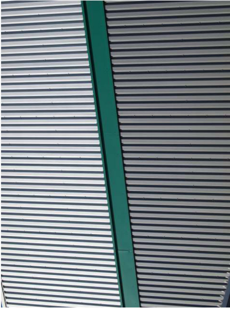
DETAIL 1 Horizontal and vertical recessed contrast colour flashing (grey/silver proposed)
