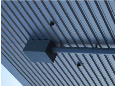
DETAIL 4 External rainwater goods in contrast colour
